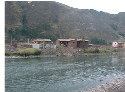
Details of the buildings trying to gain ground in the floodplain downstream right bank.
