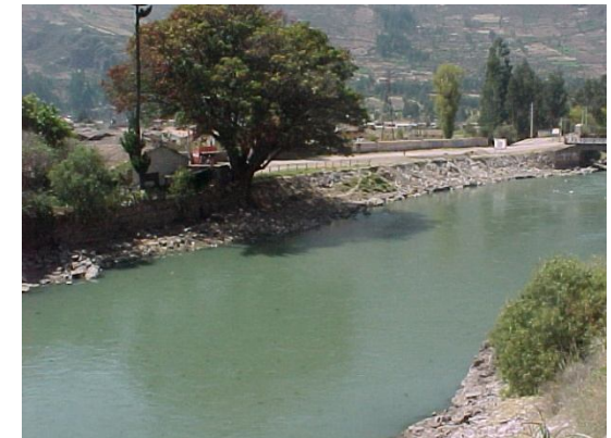
Temporary protective wall built by the homeowners who do not meet necessary conditions for their protection.
