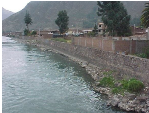
Contention wall that protects part of the right bank of the river Vilcanota.
